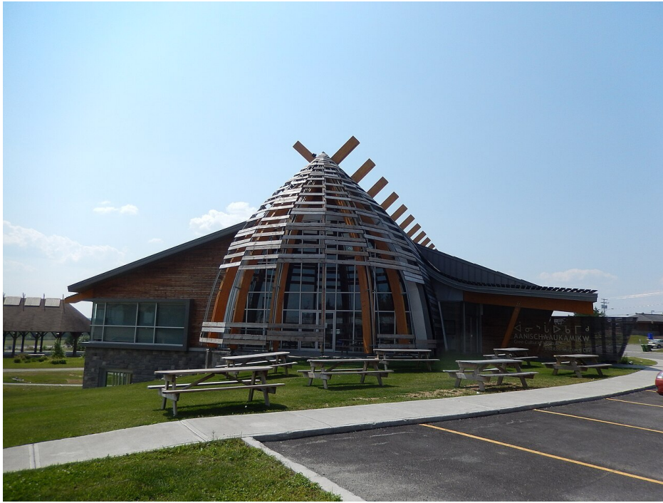
Figure 1. Aanischaaukamikw Cree Cultural Centre (2011) designed by architect Douglas Cardinal through a series of visioning sessions and close collaboration with Elders and Rubin Rotman Architects of Montreal. (Ouje-Bougoumou, Quebec). Fralambert. (2014). Copyright: Oujé-Bougoumou en août 2014. [online image]. Wikimedia Commons.
